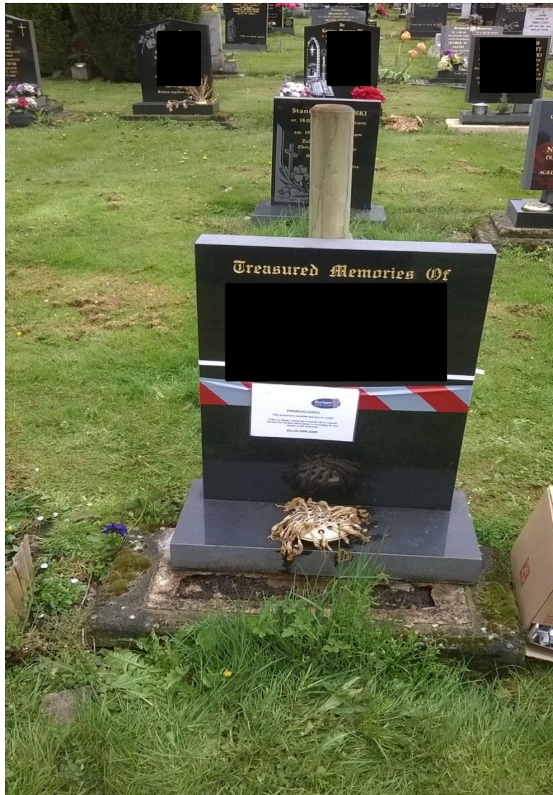
Example of a warning tape notice and banding attached to an unsafe memorial.
