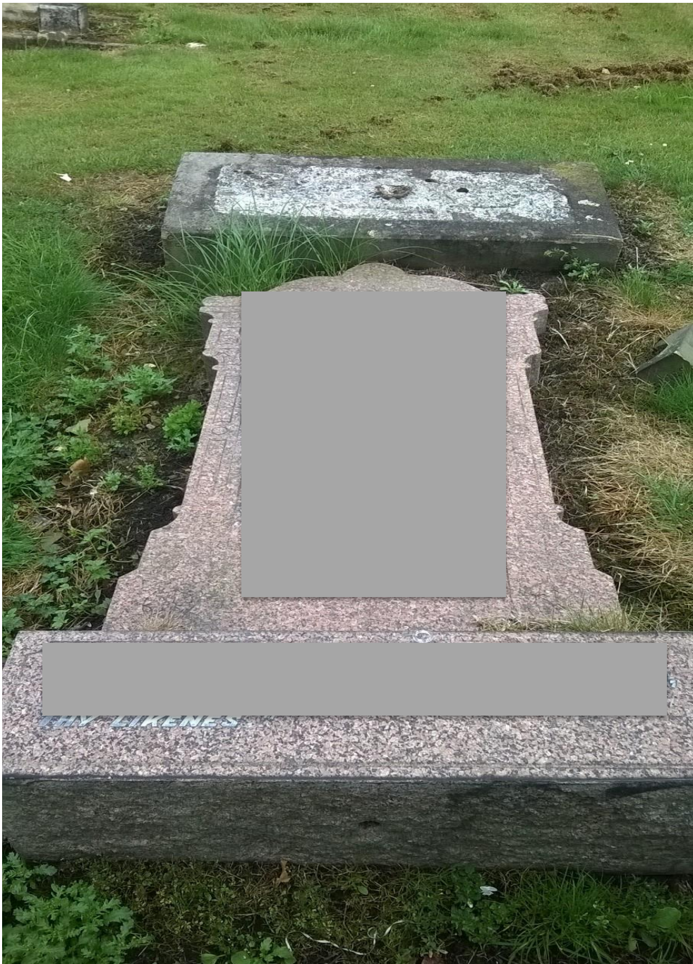
Example of an unsafe memorial, with no dowels, laid flat on the existing grave space.
