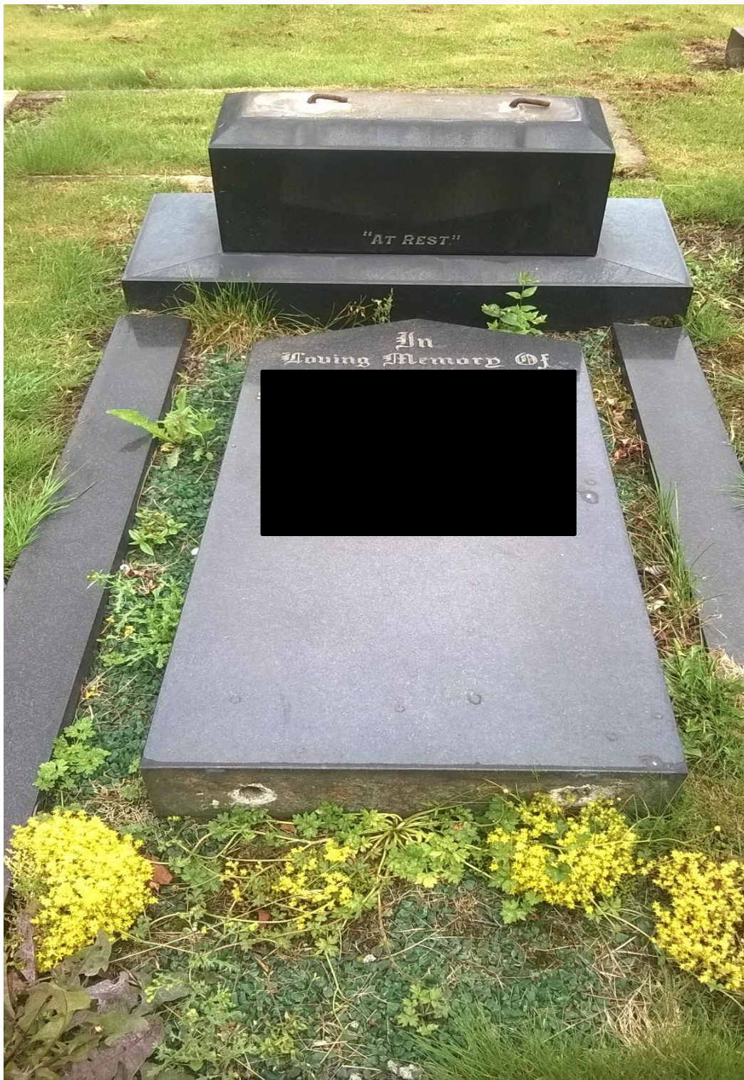
Example of an unsafe memorial laid flat in between existing kerb sets.
