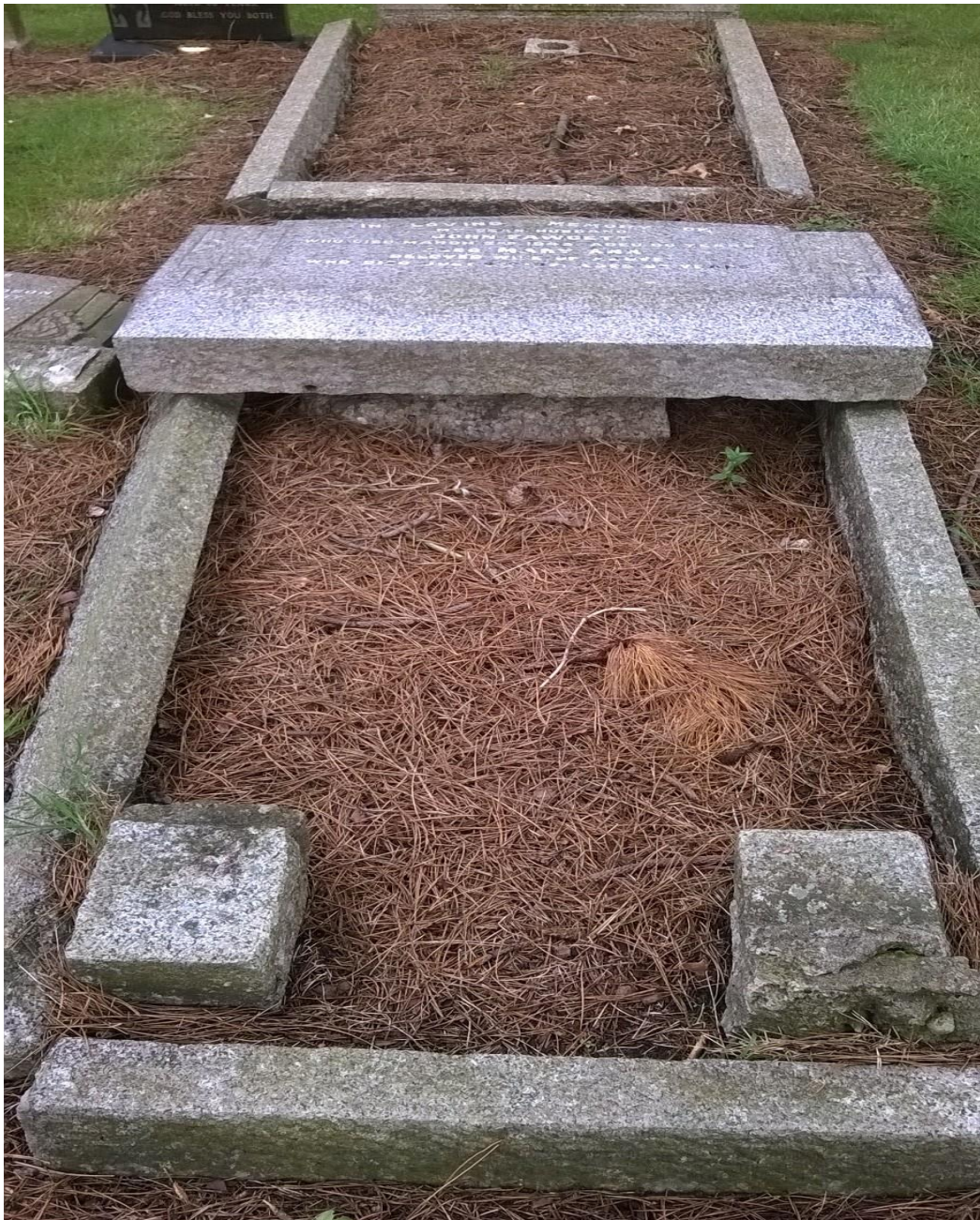
Example of an unsafe memorial laid flat on the head of the kerbset.
