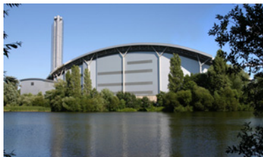
Lakeside Energy from Waste, Colnbrook, Berkshire
