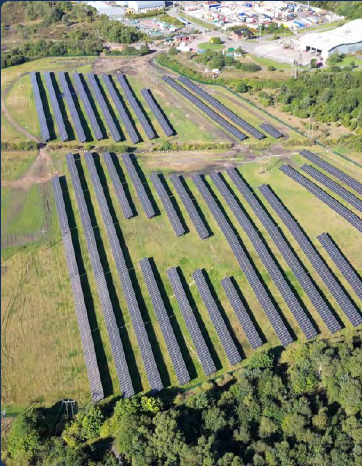
Solar farm at Annfield Plain. Part of the low Carbon Depot.
