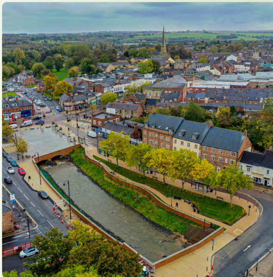
Chester-le-Street, Chester Burn de-culverting project.
