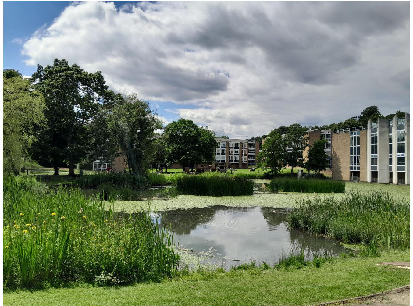
Fig 38 Van Mildert College, the 20 th century purpose built college designed to embrace the landscape that has created a leafy park land setting, with the lake as its natural focal point.
