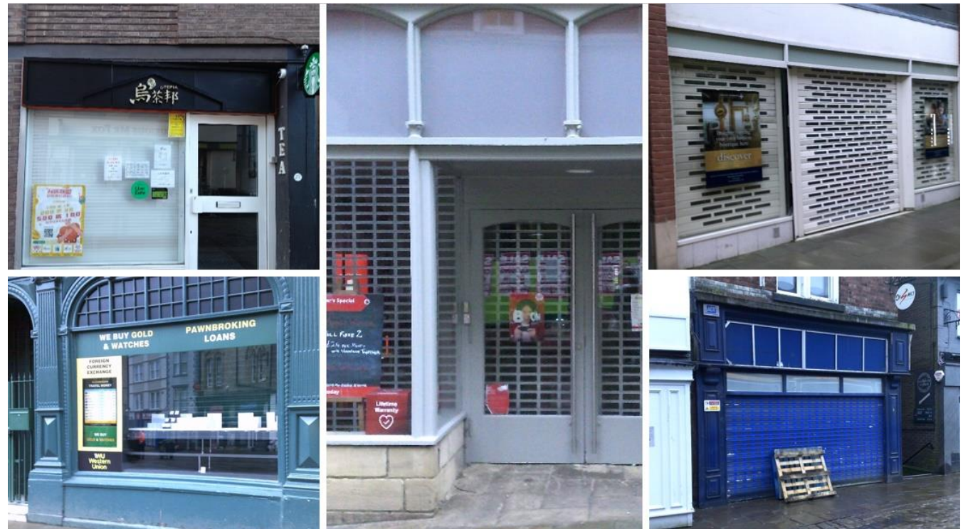
Fig 23 , above, examples of the different types of security shutters found within the city. Completely solid roller shutters should be avoided as they have the appearance of garage doors that are very out of keeping and visually incongruous giving a “deadening” visual affect. Grill and perforated types allow views through and those set well back from the shop window can be visually less impactful. The design should take into consideration the significance of the building and its role in the streetscene.
