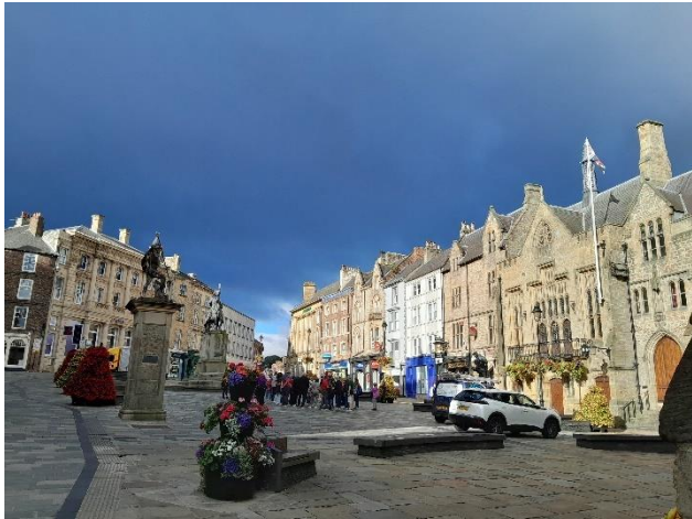
Fig 44 the medieval civic space of the Market Place and the newly created public realm at Freemans Place.
