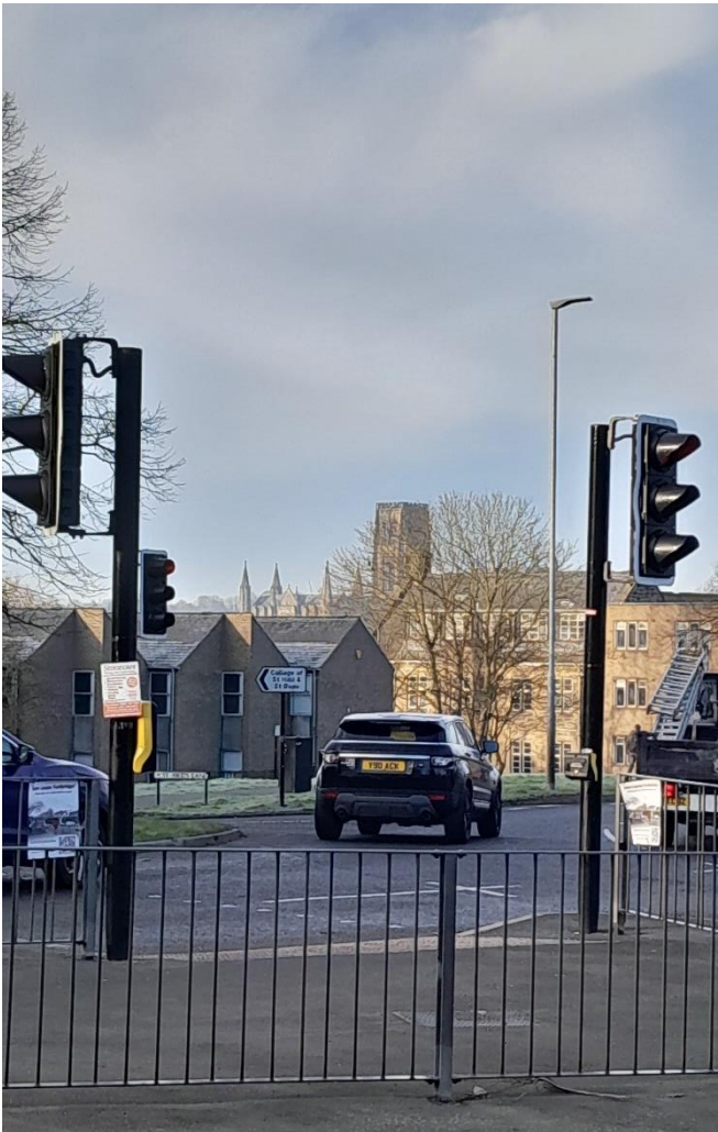
Fig 28 , the view of the cathedral from the roundabout at the bottom of Gilesgate Bank, the extent and quality of the view reduced by the modern development blocks and street clutter in the foreground.
