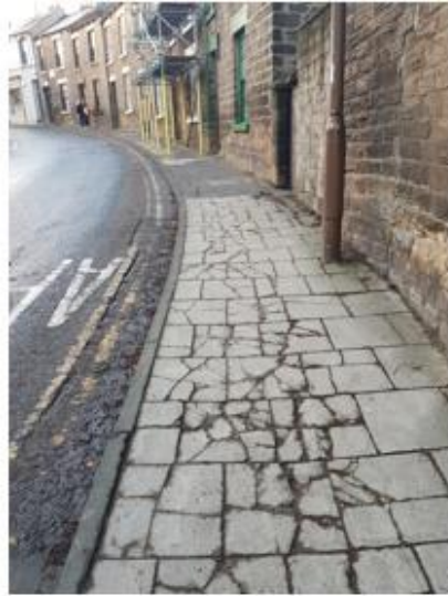
Fig 69 examples of deteriorated and poorly repaired street surfacing treatments that are commonly found across the conservation areas. Reversal of such impacts and future prevention would be highly beneficial to the character and appearance of the place.
