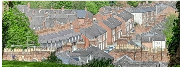
Fig 9 , an example of a typical historic terraced roofscape a familiar scene within Durham City.
