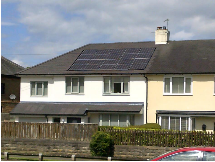
Fig 66 while still visible solar panels integrated into the roof plain on buildings of lower character can be less impactful in the streetscene.
