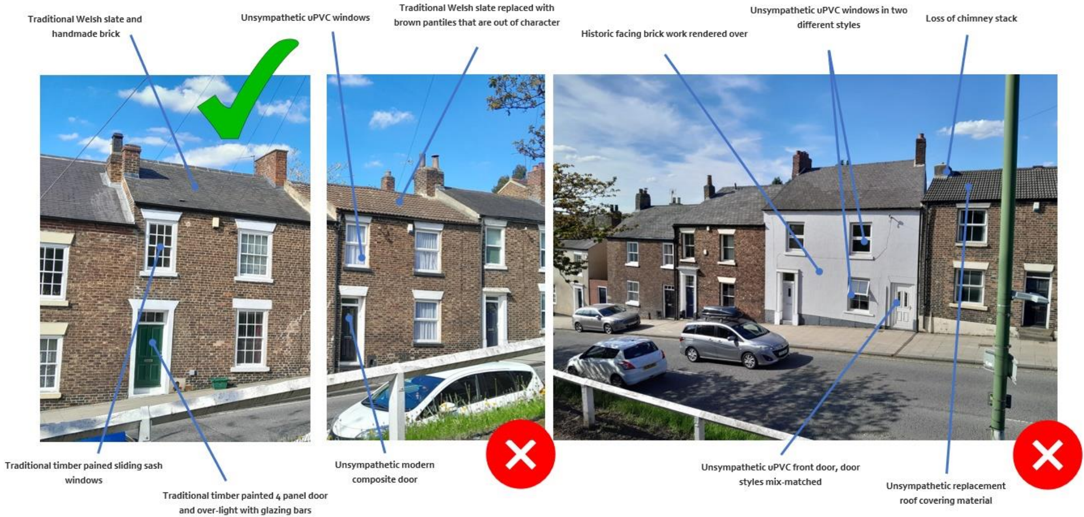
Fig 26 , streetscene views highlighting unsympathetic alterations to historic terraced properties that are commonly seen across the city.
