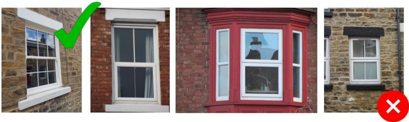
Fig 25. above an example of a uPVC heritage sash window (left) showing the different in aesthetic quality compared to standard bottom different styles of standard uPVC casement windows that fail to imitate a traditional sash appearance.
