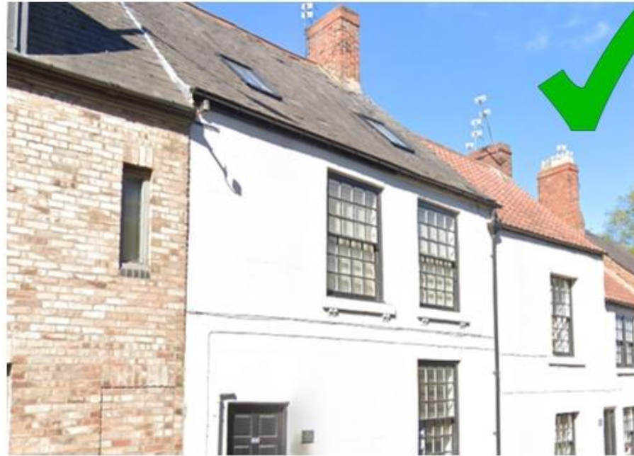
Fig 11 , example of conservation style roof lights that appear sympathetic (top), below standard roof-lights haphazardly arranged.
