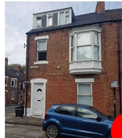
Fig 10 , an example of well-designed traditional dormer (top) and poor quality dormer in the same historic terrace.
