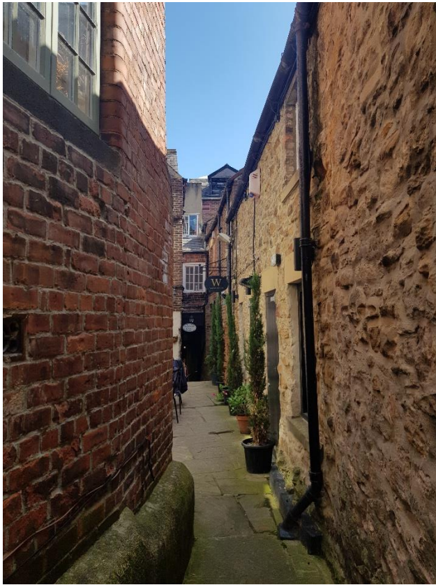
Fig 48 example of a well preserved historic vennal on the west side of Sadler Street, an inviting space of strong historic character.
