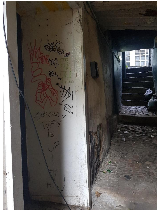
Fig 49 in contrast the historic vennal of Drury Lane on the east side of Sadler Street a very poor environment leading down to the riverside with deteriorated fabric, litter and graffiti.
