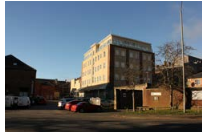
Modern residential block in the conservation area
