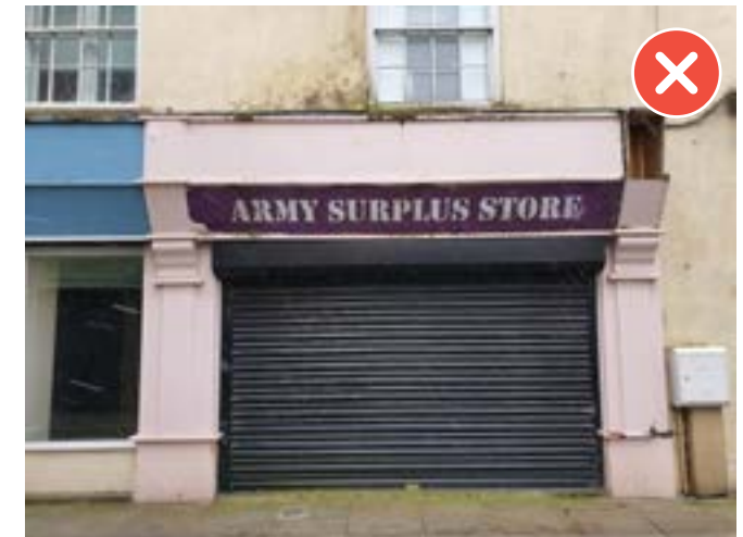
Solid roller shutters create an inactive and unpleasant streetscene when closed
