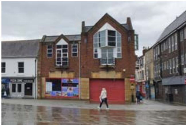
Detracting building on Market Place
