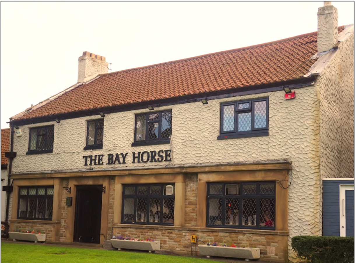
Midridge's Valued Village Assets: the Village Hall (top) and The Bay Horse Public House (bottom)
