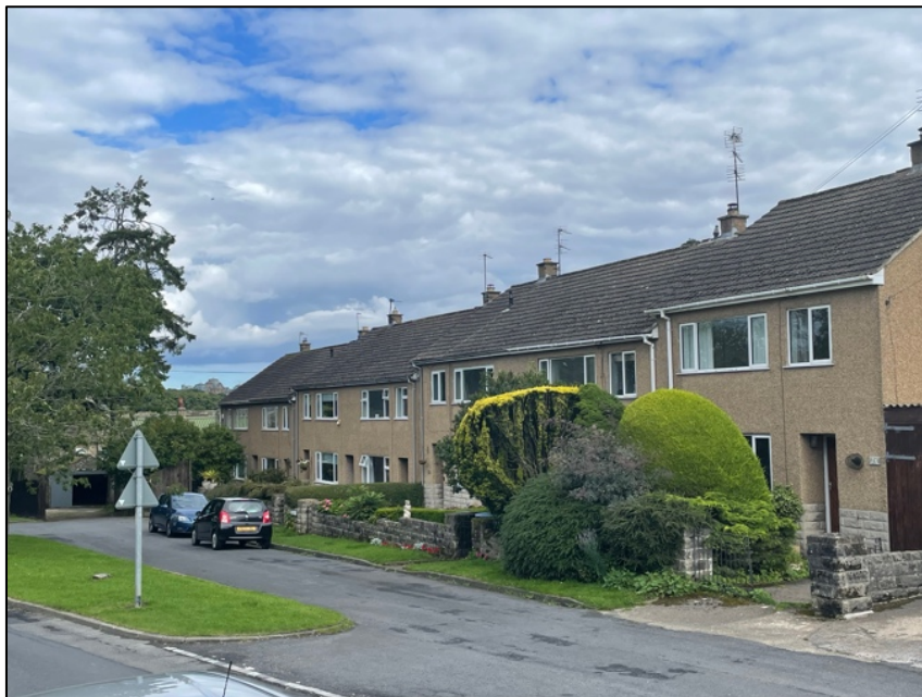
Photos 27: Terraced houses in Boldron Lane
