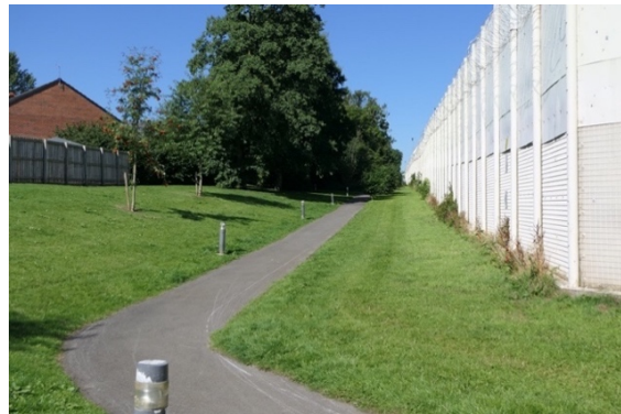
View NW of path between Grangefields & HMYOI
