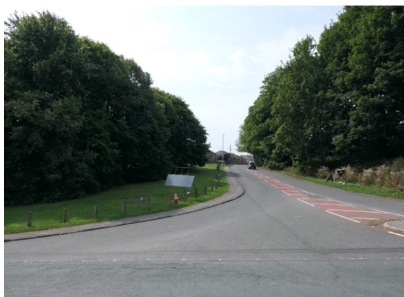
View SW of Bowes Road from Lartington Road
