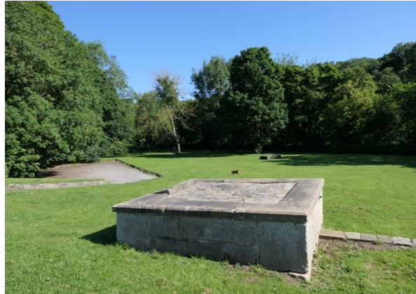
Base of former Ullathorne Mill chimney
