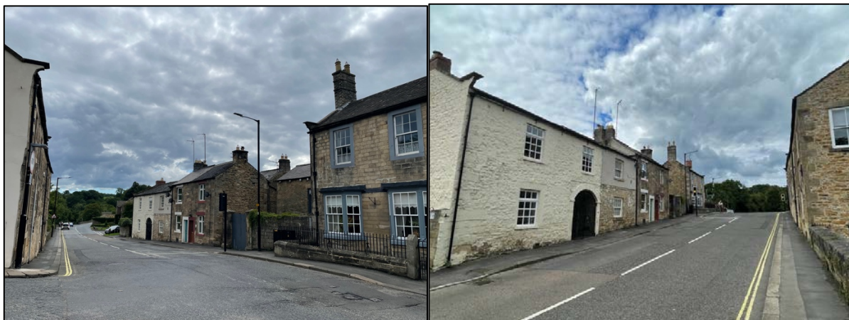
Photos 19 & 20: Bridge End
