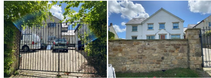
Images 37 and 38 showing new boundary walling and hard surfacing
