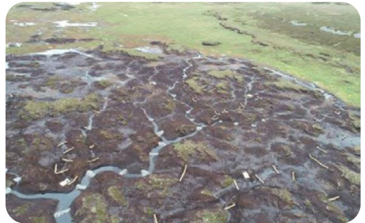
Bare peat restoration showing coir rolls and stone dams: © North Pennines AONB Partnership
