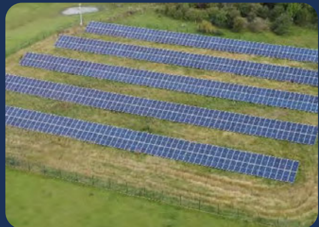
Tanfield Lea Solar Farm. A 250kW solar farm providing green electricity to a Durham County Council office building.
