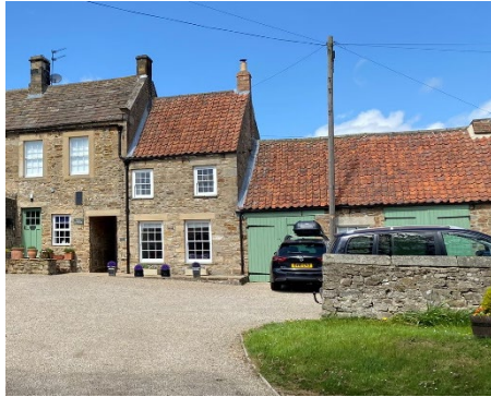
Image 10 Former Smithy and Outbuilding
