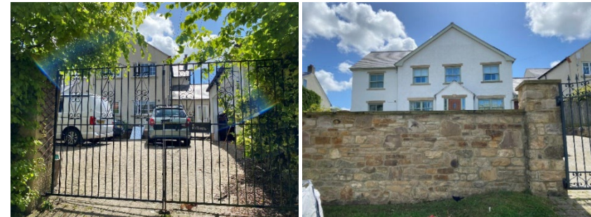
Images 19 and 20 showing new boundary walling and hard surfacing
