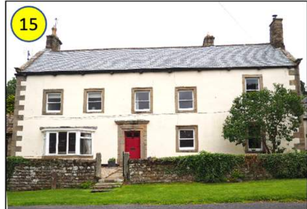
Figure 15: Traditional property with rendered front elevation, but retaining feature stone quoins, window and door surrounds
