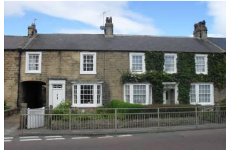
Typical roofing materials in Staindrop
