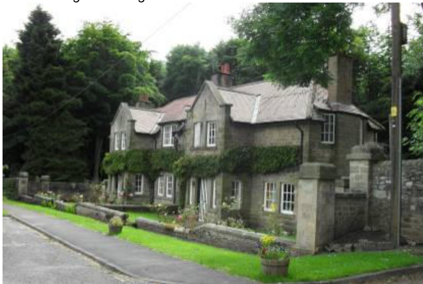
Former estate workers cottages, Raby Castle
