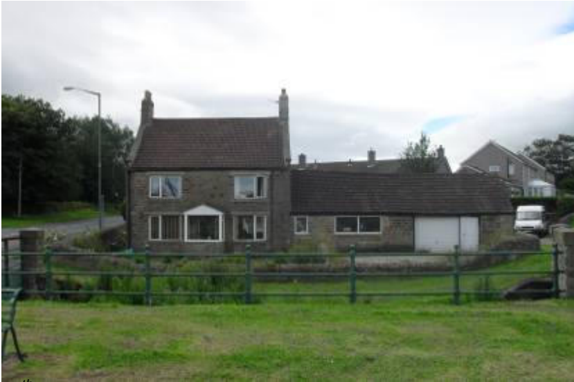
18 th century house with inappropriate detailing
