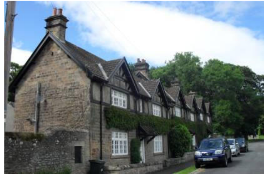
Former estate workers cottages, Raby Castle
