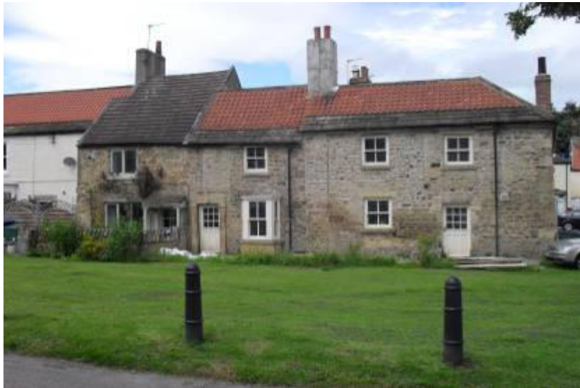
Typical roofing materials in Staindrop
