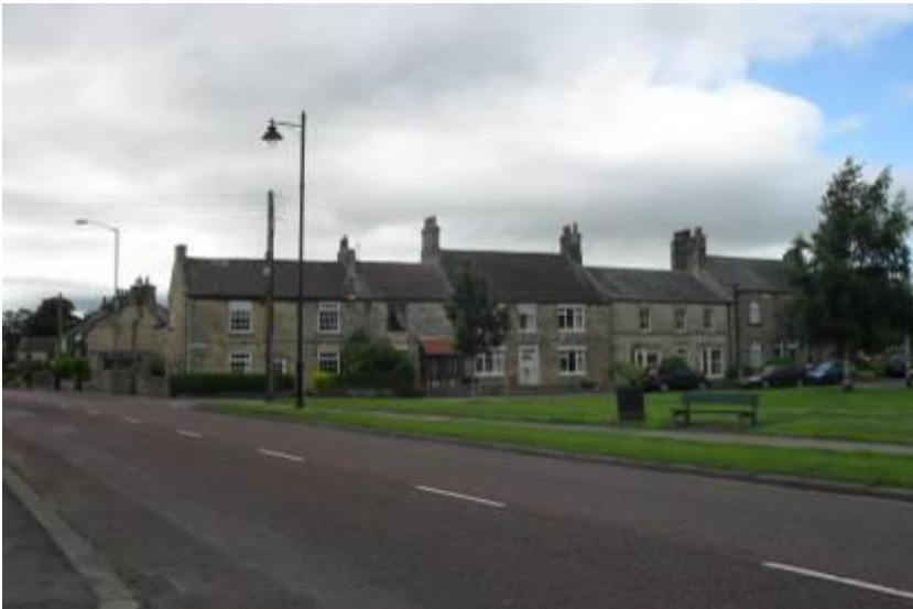
Tarmac road through village looking towards properties on North Green
