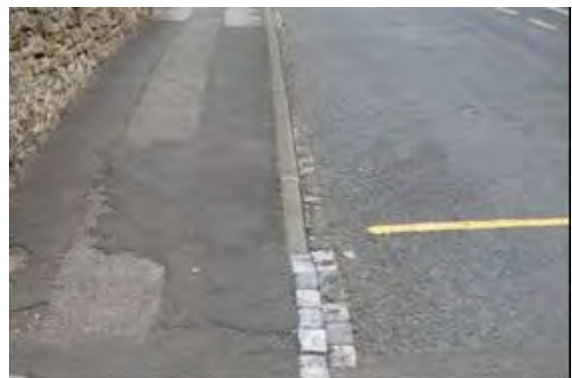
Scoria blocks often survive under tarmacadum surfaces and contribute to the interest of the area
