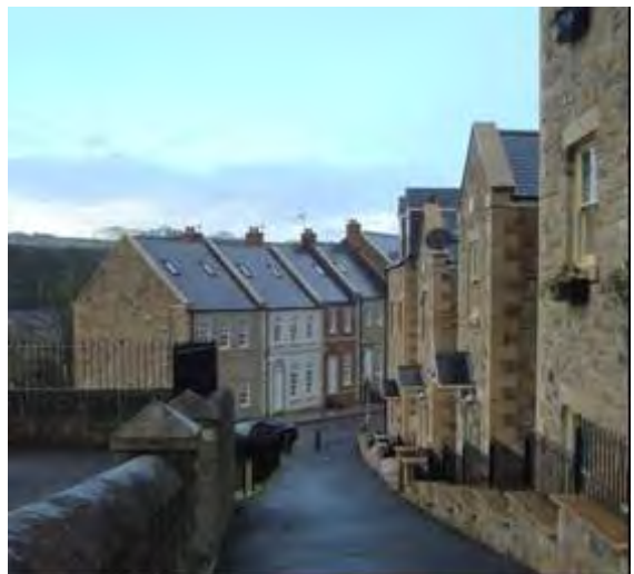
Wood Street development – buildings follow the line of the historic road pattern in this area and are well designed and detailed
