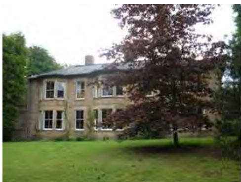
Shotley Lodge, Tinkler Hill – one of the grand residences built in the village during the mid to late 19th century
