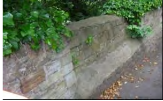
Unusual feature – a seat built into the wall on Church Bank needed for rest on the climb
