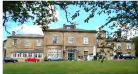
Shotley Park – built in 1842. Example of a fine classically influenced building.
