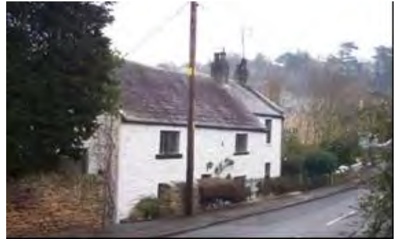
Orchard Cottage – dating from the 18th century, one of a number of cottages that line the B6278
