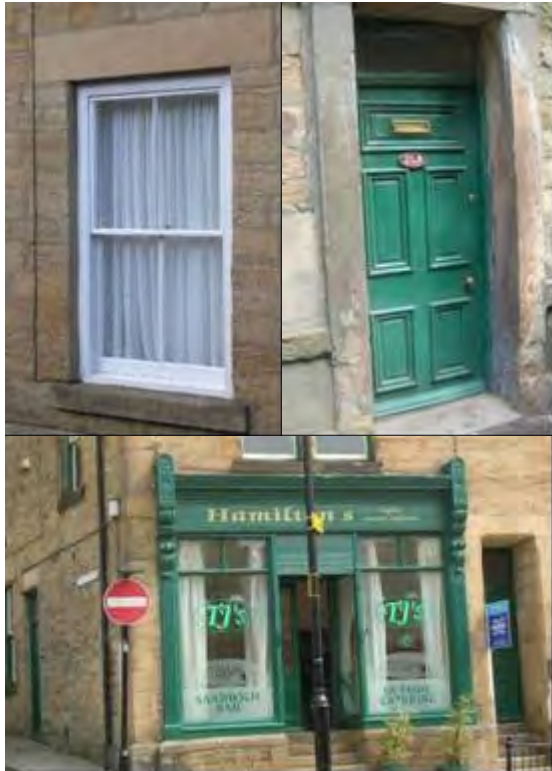
Traditional timber sash windows, panel doors and shopfronts continue to be important features of the conservation area, contributing greatly to the integrity of the place.
