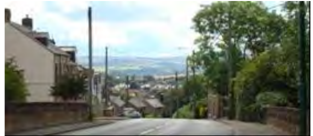
Summerhill: this forms the entrance to the village from the east and accommodates buildings that relate to the station building, which played an important role in the development of the village
