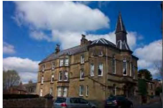
The old Town Hall, Snow's Green Road – now apartments and a nursery
