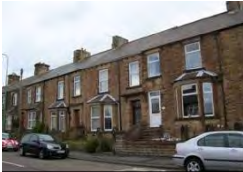
The uniform frontages of the terraces of Benfieldside Road
