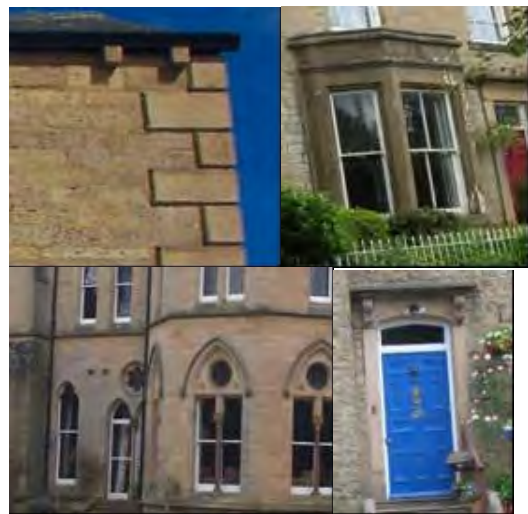
Stone detailing has been used to adorn the buildings of the conservation area. Features include quoins, bay windows, dentil courses, string courses and door and window surrounds
