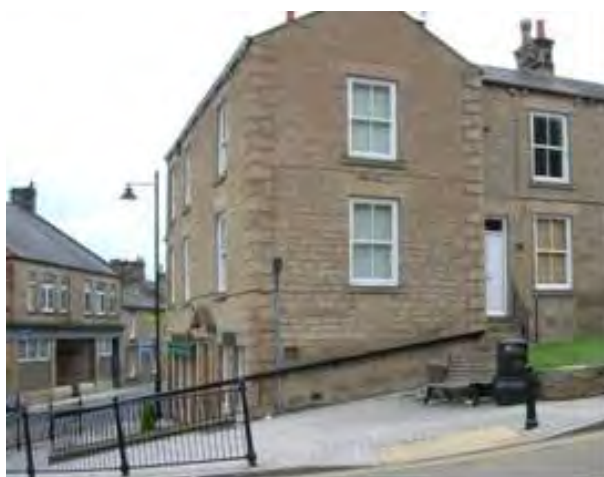
New paving and street furniture has been installed in the heart of the village as part of a recent landscaping scheme
