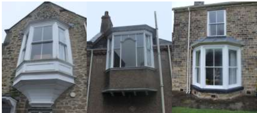
A variety of attractive bay windows.
