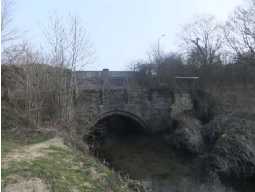
Sherburn House Bridge a Scheduled Monument.
