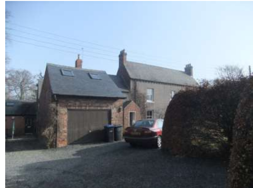
Sherburn House Farm, left the main farmhouse and above the attached single storey buildings.
