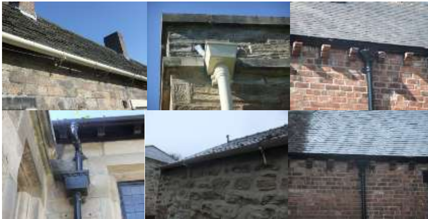
Examples of the variety in rain water goods.
