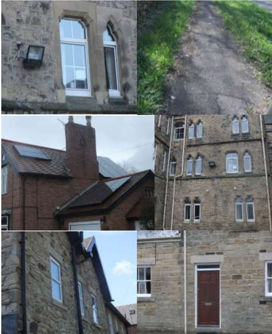
Examples of unsympathetic window and door replacements, deteriorating foot paths and prominent solar modules.
