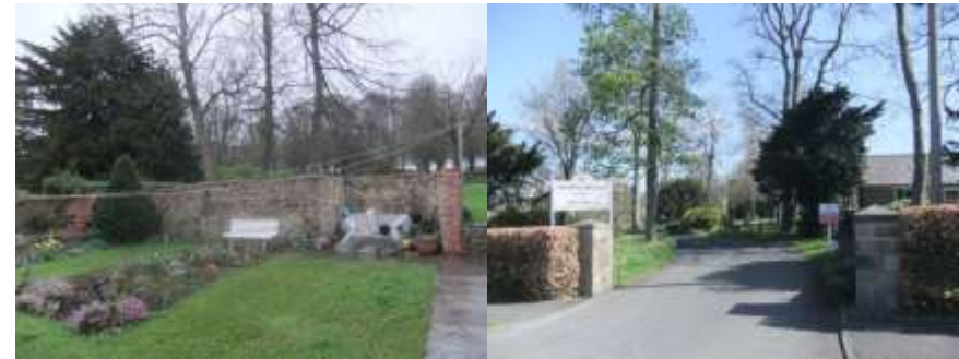
Above left, walls enclosing private gardens are also of value, and right the entrance into Sherburn Hospital flanked by stone piers.
