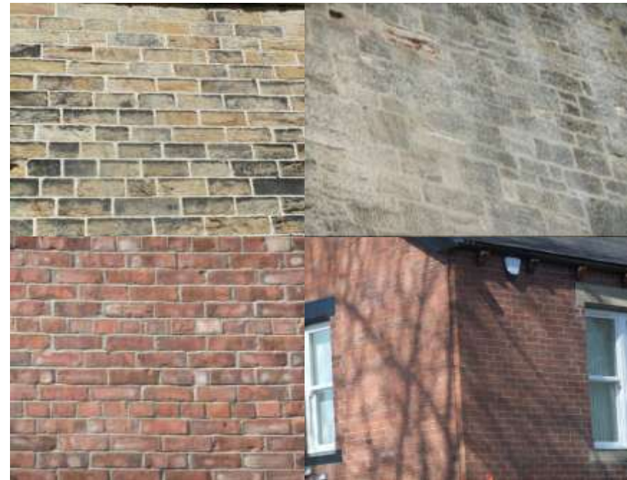
Examples of stonework and brickwork.
