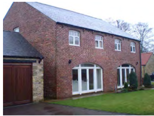
Fig 24: The Hayloft and garage a former cart shed or open shelter which has been sympathetically converted
