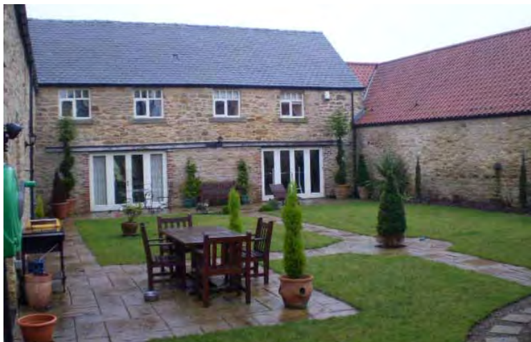
Fig 26: Priory View and the Parlour former agricultural buildings dating from the late 19C
