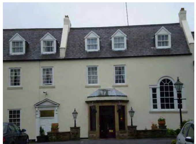
Fig 18: Hallgarth Manor Hotel, front elevation, the Venetian stair window is to the right
