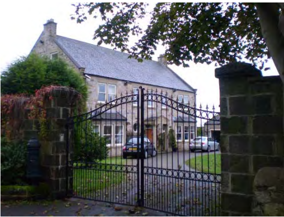
Fig 14: Hallgarth House dating from the mid to late C20
