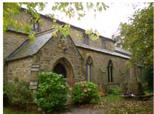
Fig 10: The main entrance to St Laurence's Church
