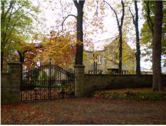
Fig 13: The Old Vicarage constructed in 1833
