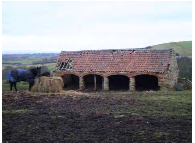
Fig 4: The single-storey cart shed, a historic building demarcating the main entrance into the village.
