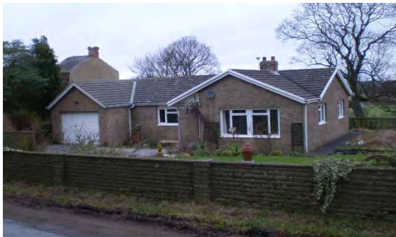
Fig 6: Tunstall Cottage a modern bungalow facing Grange Farm.
