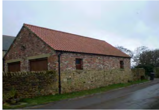
Fig 12: The detached double garage is of a traditional appearance and has been constructed from materials salvaged from the original barns.
