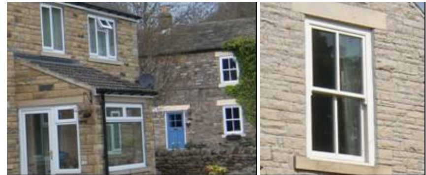
Modern windows in a modern house and a traditional style in a new extension
