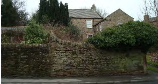
Boundary walls around The Old Rectory, Front Street – a crucial element of the character of Ebchester
