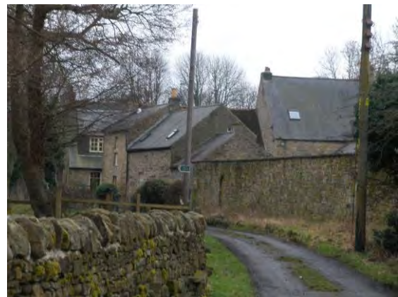
Lane Head, Mill Lane – the buildings have been constructed right up to the edge of the road, set in open countryside
