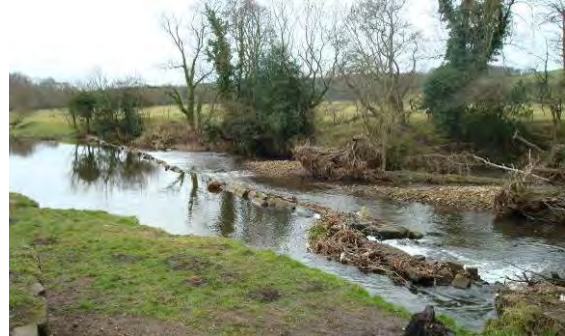
The weir of the River Derwent – the river is a visual element of the village, particularly at the bottom of Chare Bank.
