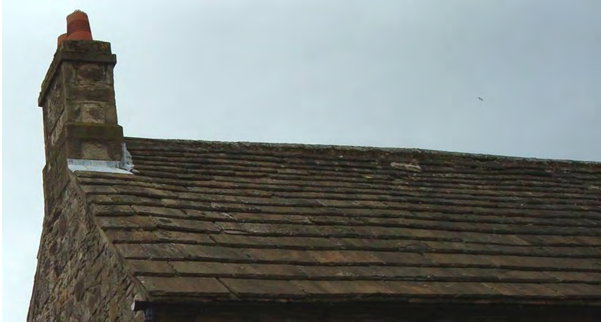
Stone slab roof of Jubilee House – a rare example of a local roofing tradition
