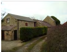
(9) Outbuildings to Mains Farm, Front Street Collection of random rubble stone outbuildings of 2 and 2½ storeys in height. Stone lintels and cills to characteristically
