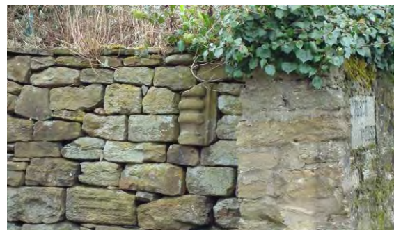
Reused stones in the wall to Church House
