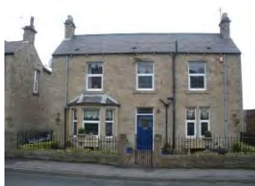
(13) Poplar House Early 20 th century double fronted house, constructed of squared stone to front elevation and rubble to side and rear, with quoin details
