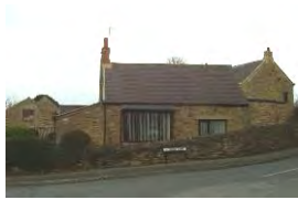
(8) Mains Cottage, Front Street Pre mid 19 th century farm cottage. Constructed of stone rubble with a Welsh slate roof.
