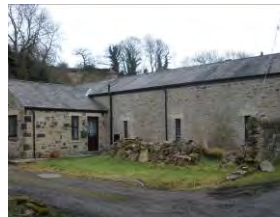
(16) The Stables Single storey stone building, converted to residential use from an old outbuilding to Ebchester Corn Mill. Has characteristically small openings with a slate roof.
