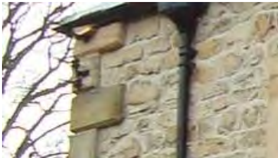
Stone quoins are used to define the corner of buildings – this is a rare example of a raised quoin detail
