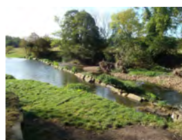
(18) The weir The weir is constructed of sandstone. A weir has been in this location for many years and it is marked on early Ordnance survey maps.
