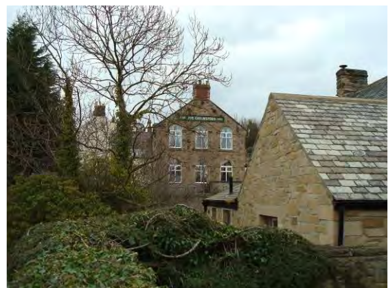
The Chelmsford – a commercial property in what is predominantly a residential community
