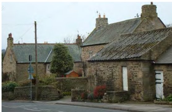
Demesne Farm – buildings of Front Street are generally set back from the street and are orientated to face the road. The space is defined by stone walls and many have associated outbuildings
