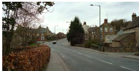
View along Front Street – views along the road taking in its built form are important, in places they offer little insight into what lies beyond
