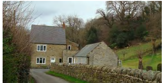
Mill House, Mill Lane – once part of Ebchester Corn Mill and the only surviving standing structure of the village's mills
