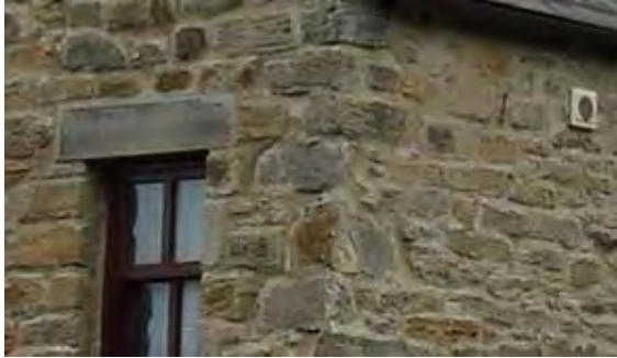
Random rubble stone construction is common in the conservation area
