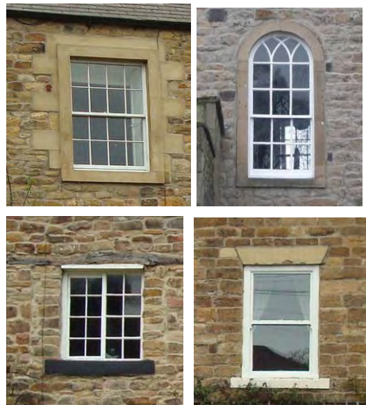
Traditional timber sash and Yorkshire sash windows set in plain stone surrounds or with stone lintels and cills continue to form part of the character of the conservation area
