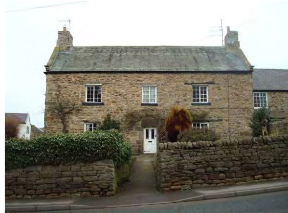
Demmesne Farm House—typical of the vernacular style of architecture that characterises Ebchester
