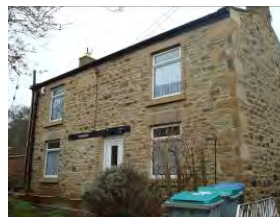
(17) No. 1, Rectory Lane Pre mid 19 th century double fronted house constructed of stone rubble with quoins to corners. Stone lintel and cills to openings.
