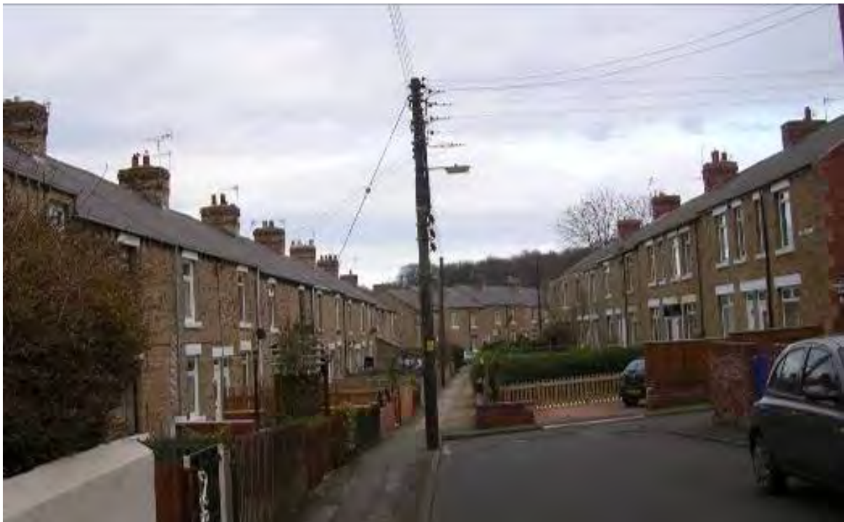
Park Terrace and Park View – turn of the 19 th / 20 th century stone terraces that contribute to the character of the core of Burnopfield
