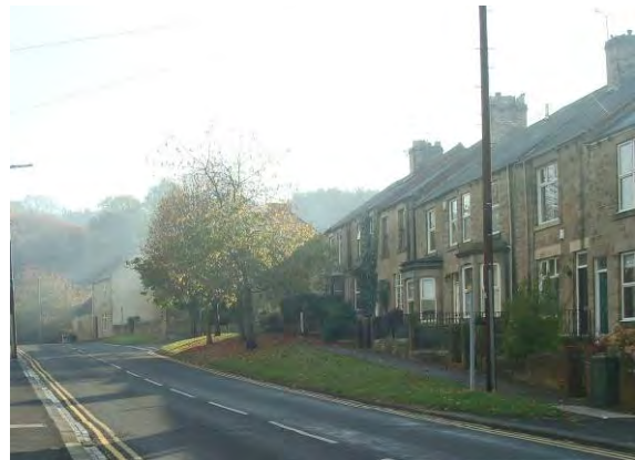
Derwent View, Front Street – the grass verge and trees soften the image of the road
