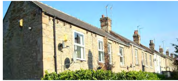
Chapel Avenue – the front elevations are cluttered with alarm boxes and satellite dishes
