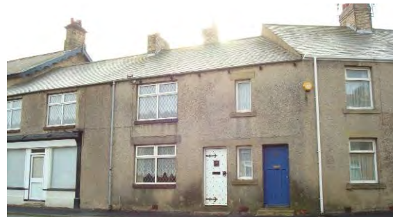
Some properties have been rendered, which serves to undermine the uniformity of the use of stone
