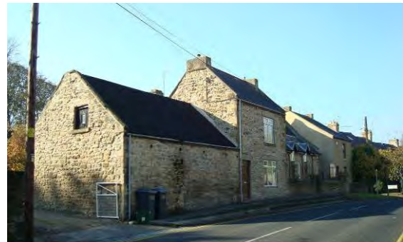
6 Front Street – an example of a simple vernacular structure that characterise this part of Burnopfield
