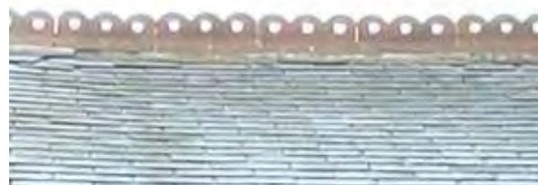
Slate creates the distinctive roofscape of the conservation area. In some instances, terracotta ridge tiles were used to add interest
