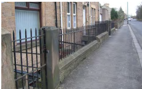
Grove Terrace – traditional railings on top of low boundary walls, typical of this character zone
