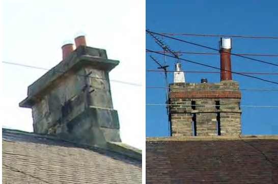
Chimney stacks constructed of stone, red or buff brick are an integral part of the design of buildings
