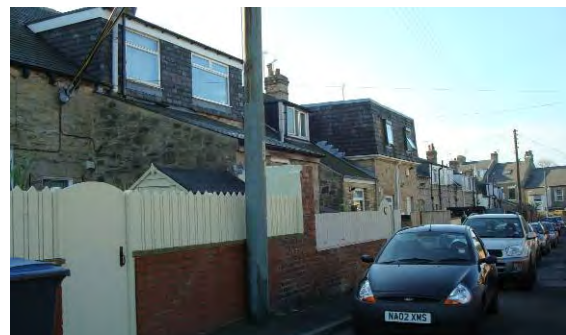
The rear elevations of Chapel Avenue have a mismatch of extensions and alterations
