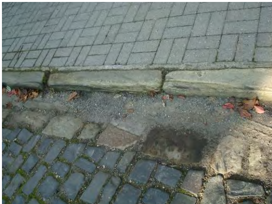
Granite setts and stone kerbs on Co-operative Terrace
