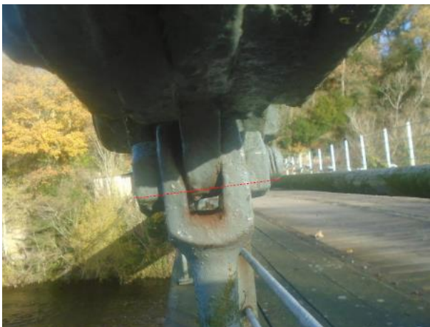
Image 3 - Typical indication of wear to other hanger/chain connections
