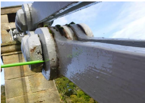
Image 6 - Deformation to chain link pin
