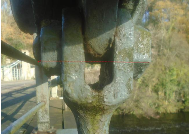
Image 4 – Typical indication of wear to other hanger/chain connections
