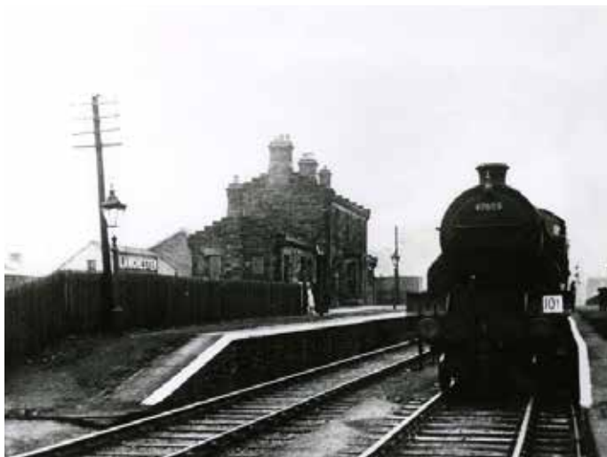
Station House and train
