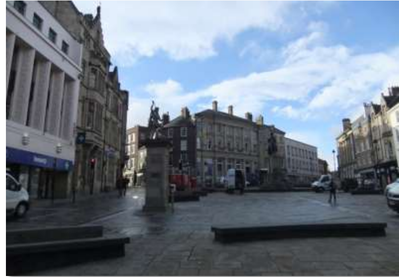
Image 10 Part of the medieval infrastructure of the city including the Market Place and the entrances to Saddler Street and Silver Street
