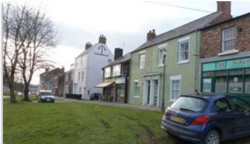
Image 33 Vehicle damage to Gilesgate Village Green
