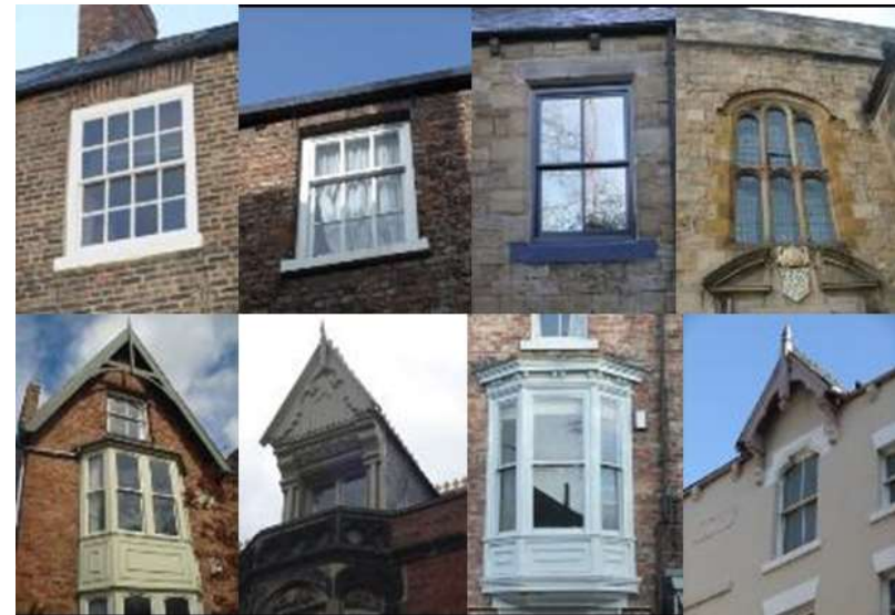
Image 13 A selection of windows from the conservation area including 16-pane and 4-pane sliding sash, Victorian bays and a decorative dormer
