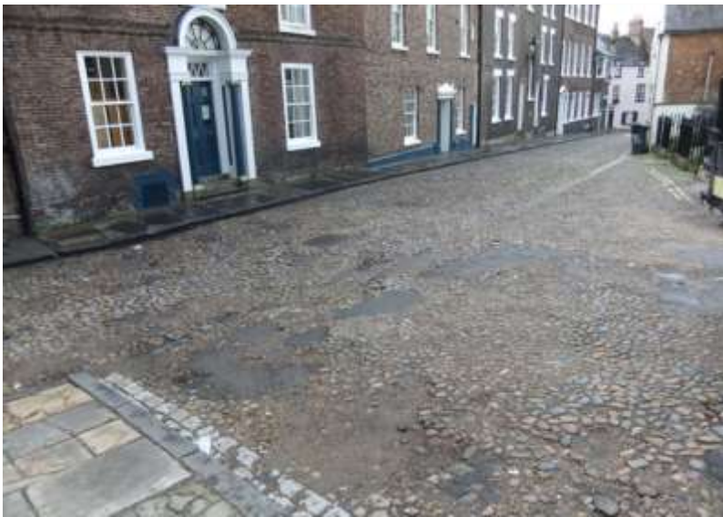
Image 31 Insensitive patch repairs to historic floorscape
