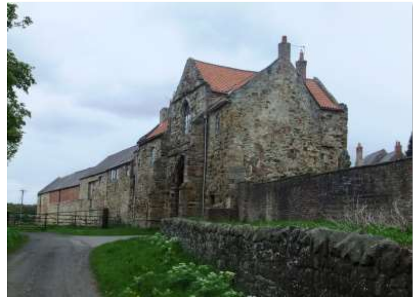
Image 81 Kepier and its Grade I gatehouse
