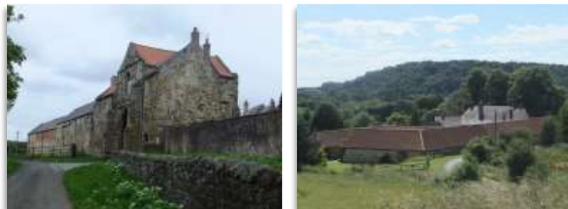
Image 4 St Hild and St Bede College, Kepier Hospital and Old Durham Gardens
