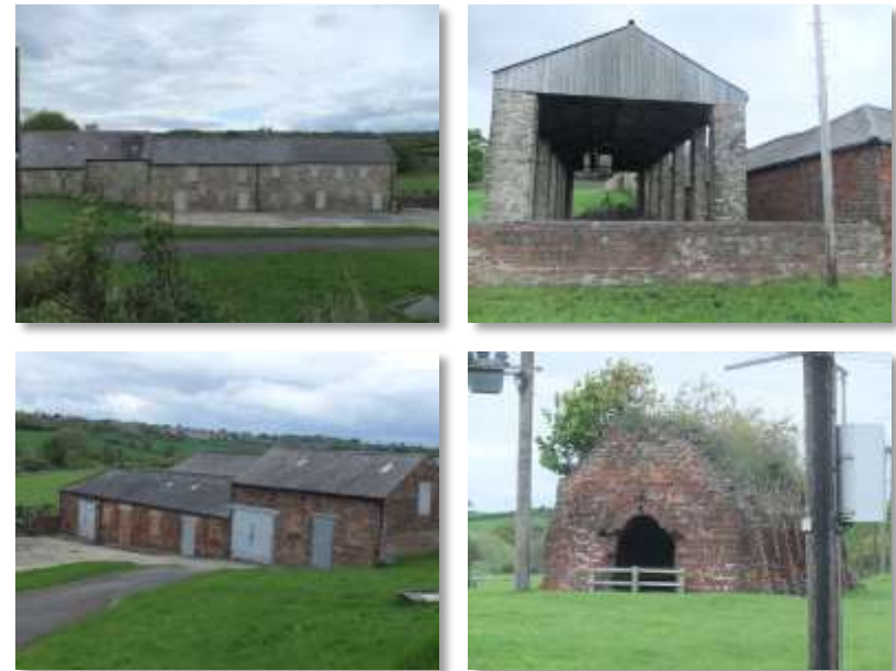
Image 83 Barns and historic brick kiln
