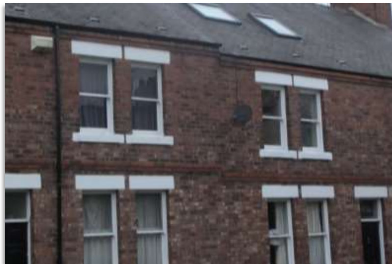
Image 72 uPVC replacements erode the original character
