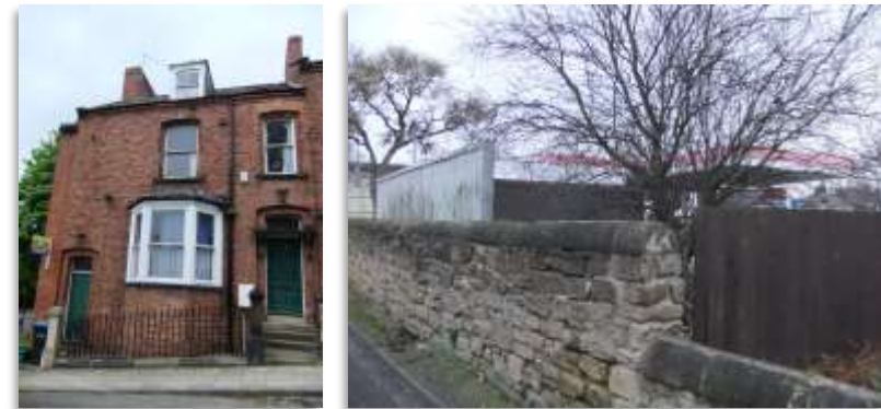
Image 39 Domestic railing and historic wall
