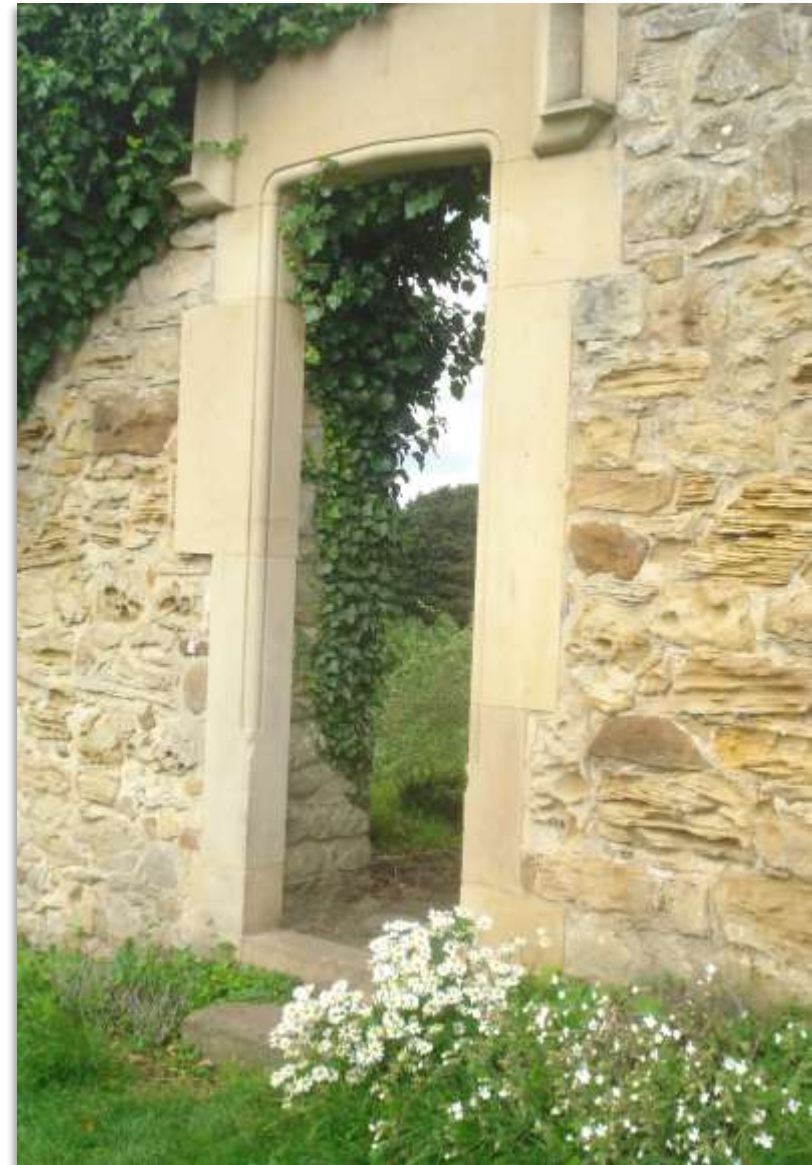
Image 13 Restored doorway to Old Durham Gardens
