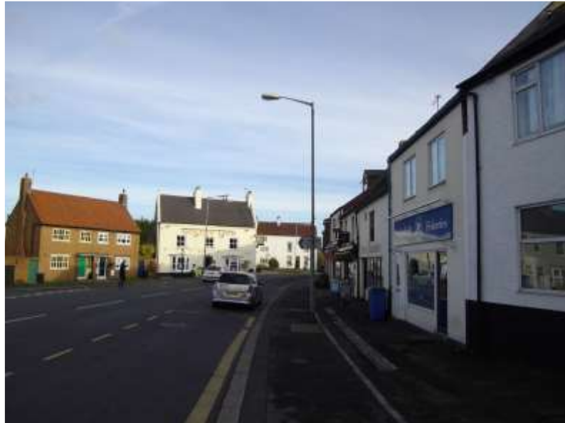
Image 33 Poor paving quality
