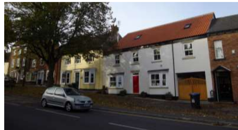
Image 10 Parish Hall above and the recently refurbished No. 31
