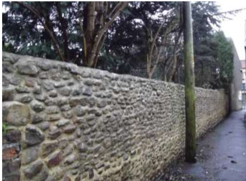
Image 17 Stone boundary walls
