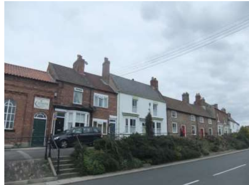
Image 51 Elevated West End
